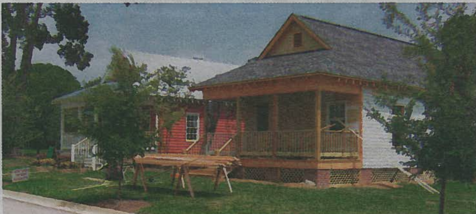
New construction at Plein Air in Taylor
